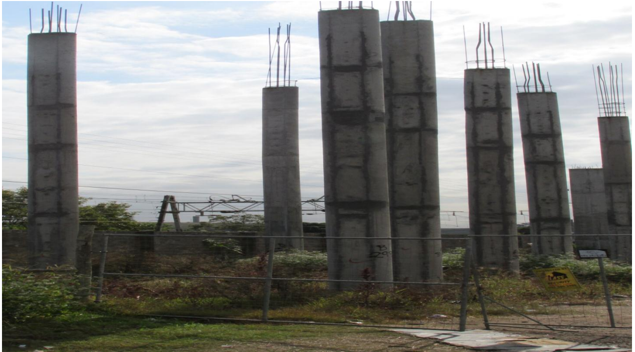
Figure 4.9: Columns that were notably cockeyed throughout the site (Source: Van Eeden, 2015)
